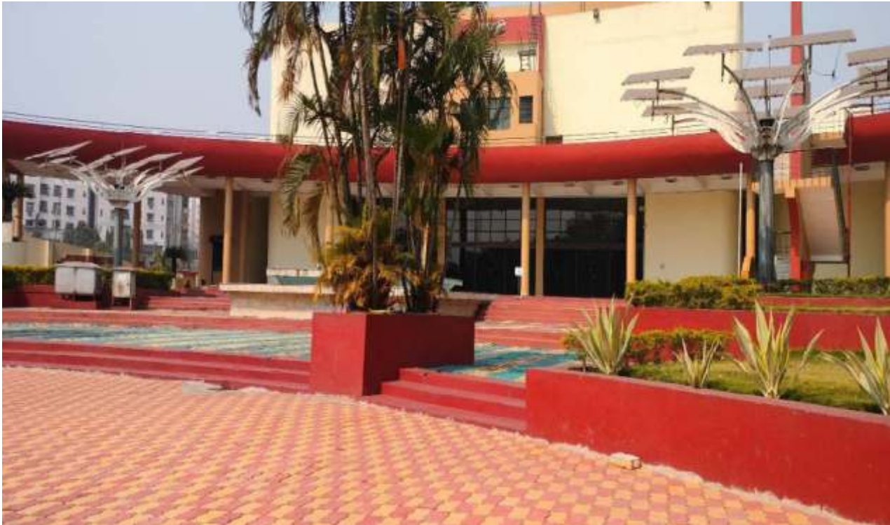
Figure 5.14: Solar Panels at a Public Auditorium in Durgapur
